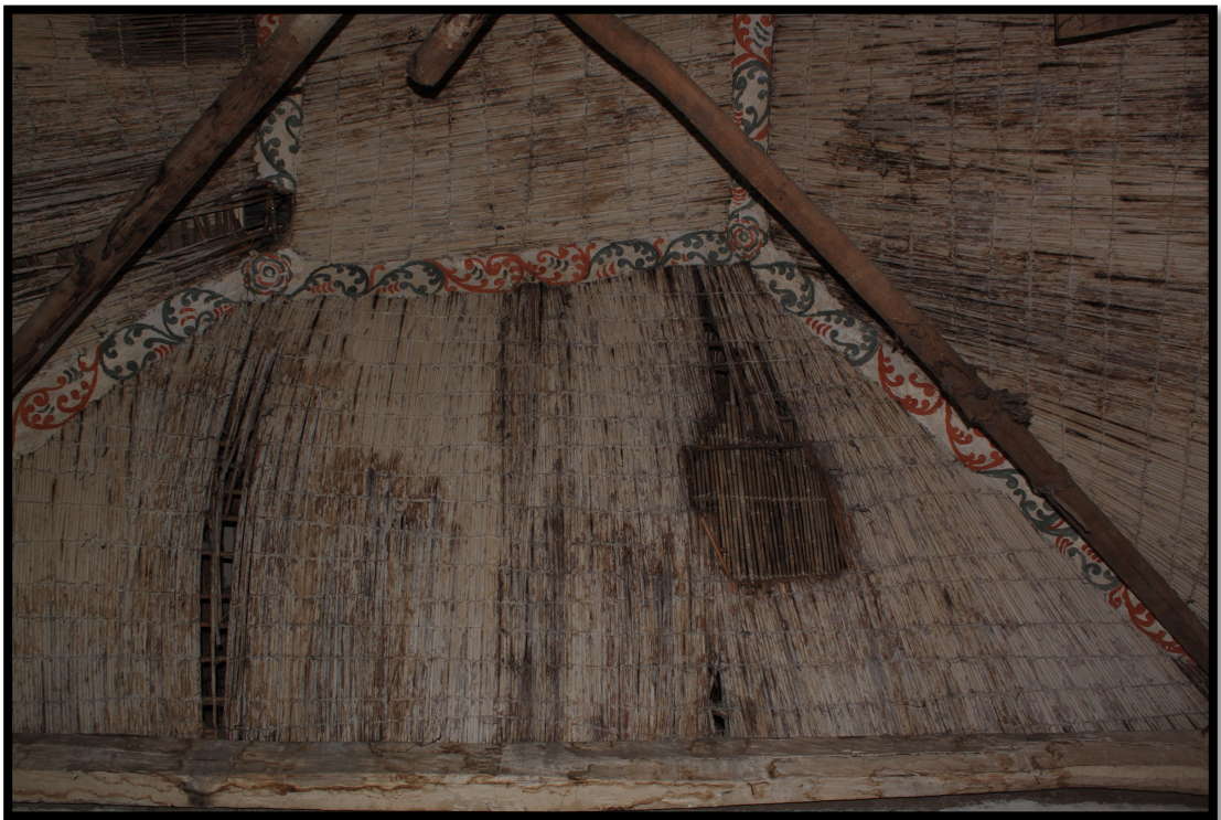
Figure 4.14. Up: Chusque and pajonal cord ( cuan ). Author's image, refurbishing process of the 16th century convent of Santo Domingo, Tunja, 2017. Down: cuan net as part of the roof in a sixteenth-century house. Author's photographs
