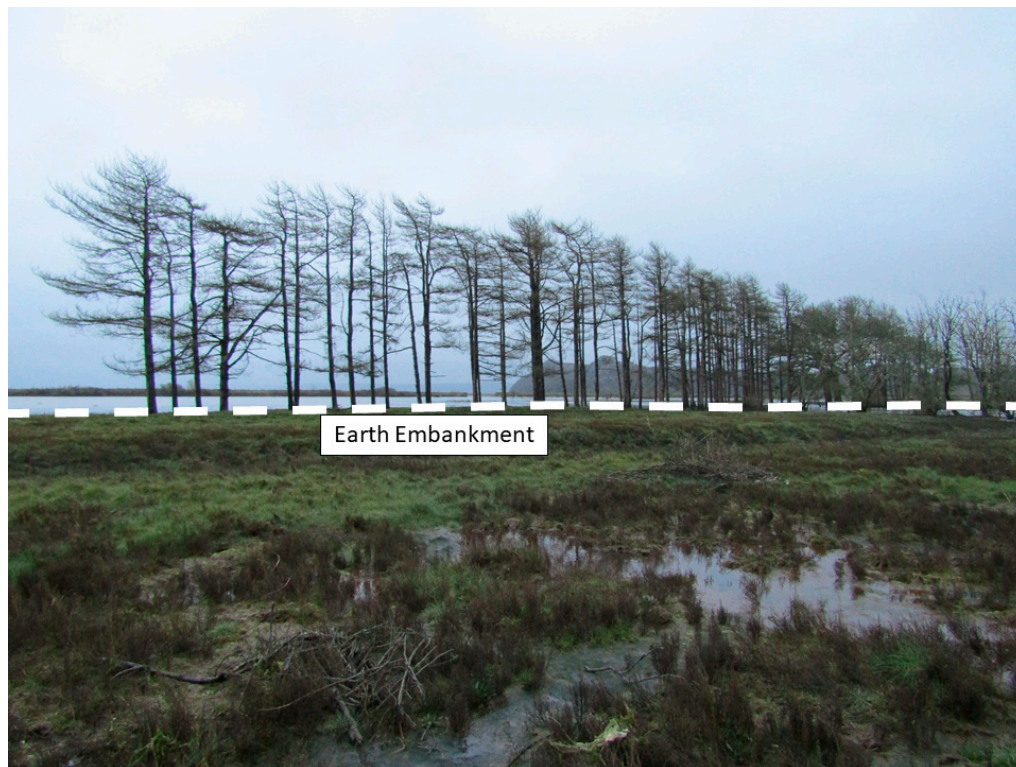
Figure 3. The tree-lined earth embankment which divides Zone 2 from Zone 3, marked by the white dashed line and labelled. The photograph was taken looking south-east towards the breach area across Zone 2 into Zone 3 (photography: H. Burgess).
