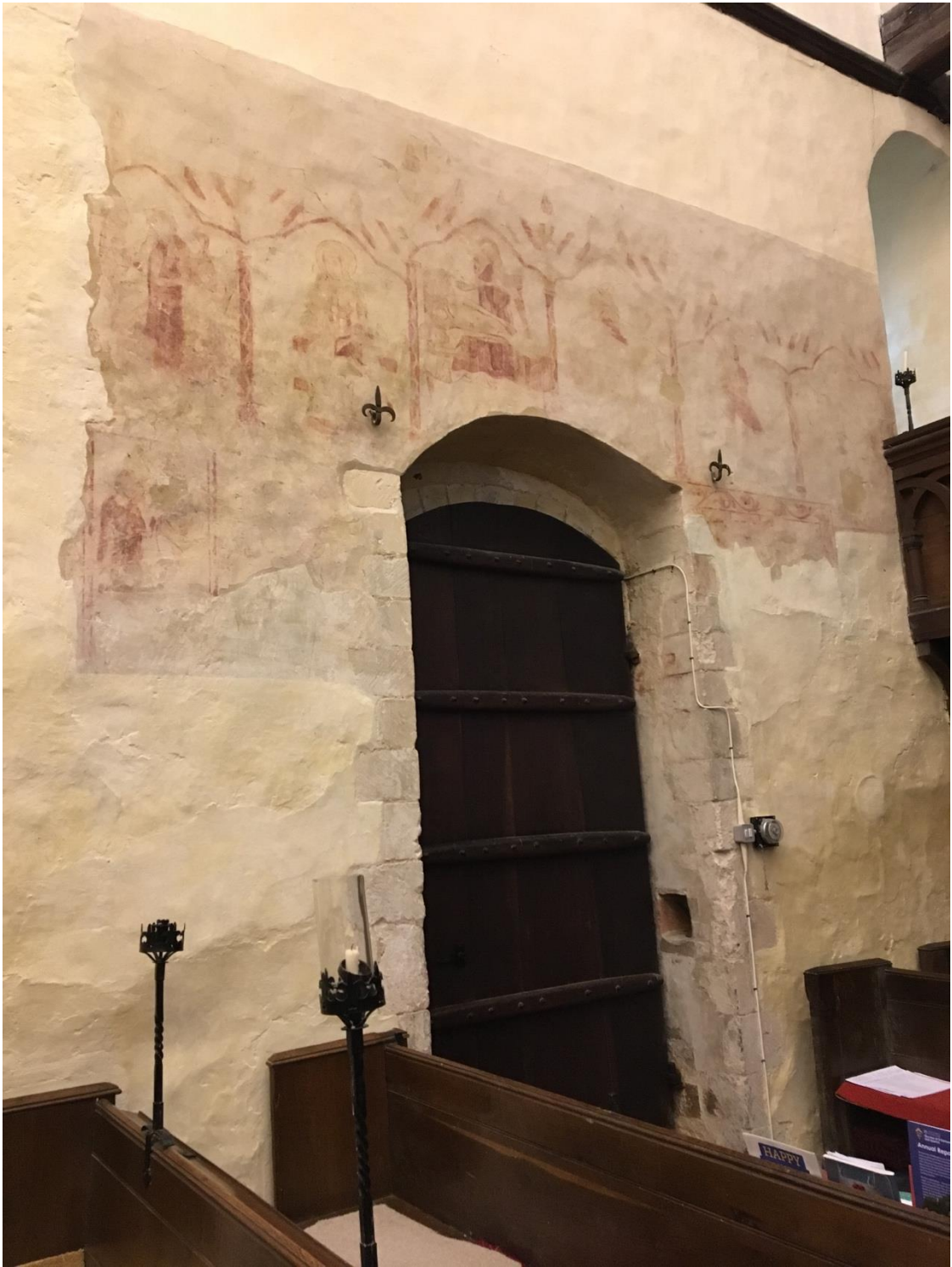
Figure 2.37b: St Mary the Virgin, Wiston (Wissington), Suffolk. Nave south wall, south door. Infancy Cycle on upper tier of paintings, St Margaret paintings on lower tier.
