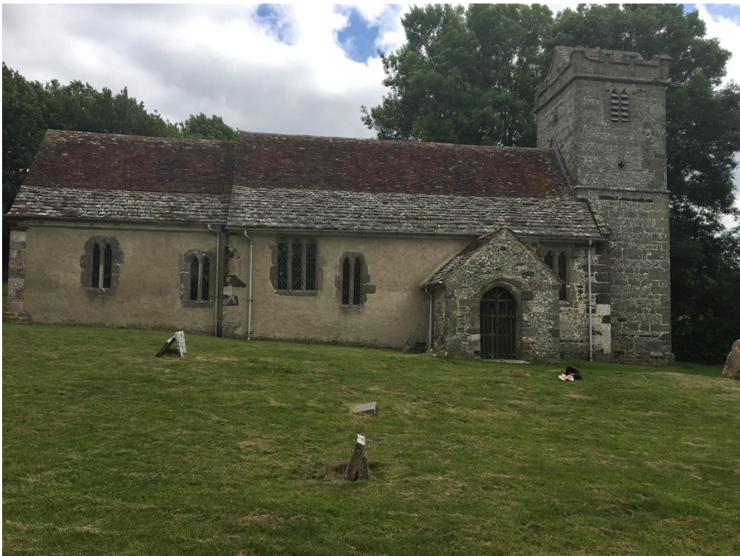
Figure 1.2: St Mary the Virgin, Tarrant Crawford, Dorset. Exterior. View of the north face of the church, north door and tower.
