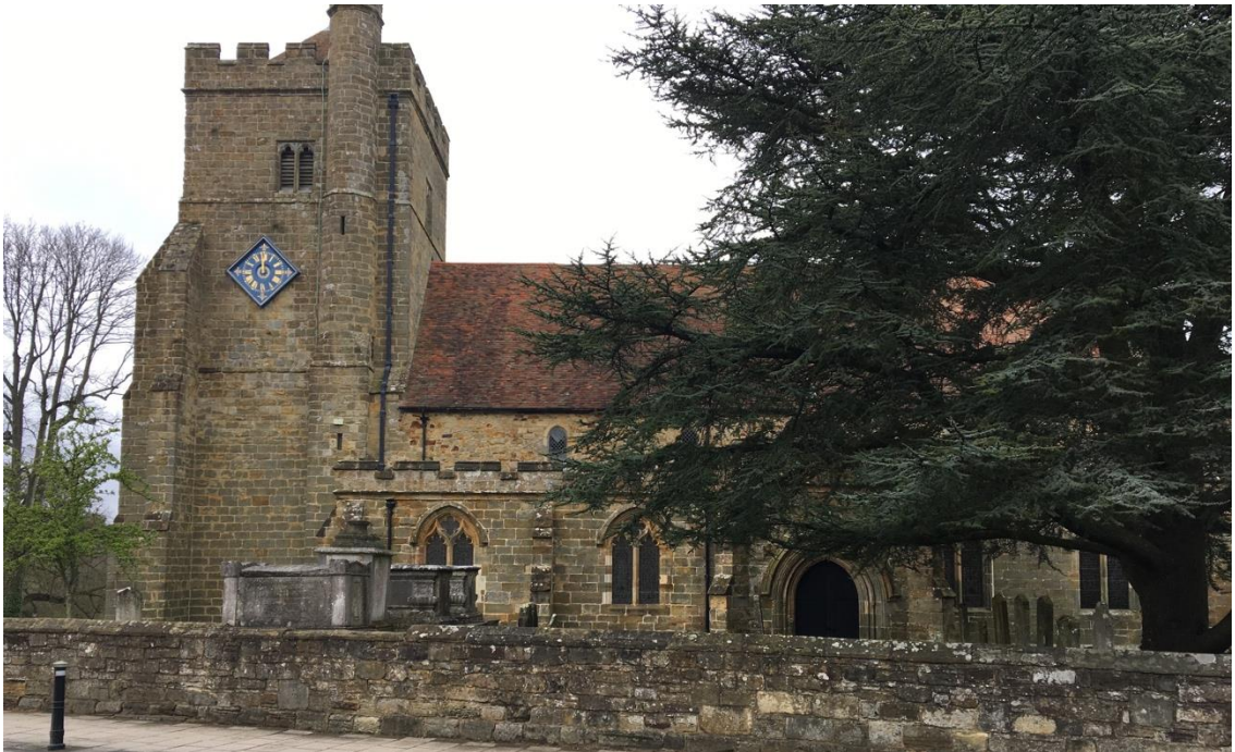
Figure 1.1: St Mary the Virgin, Battle, Sussex. Exterior. View of the south face of the church, south door and tower.
