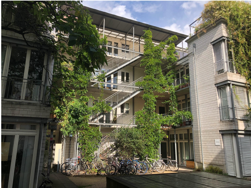
Figure 5 (left): External view of the scheme on Hellmutstrasse in Zurich, showing how the open access stair and shared balcony walkways enable various access arrangements (author).
