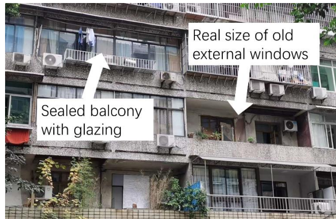
Figure 5.7: The real size of external windows in an old urban residence
