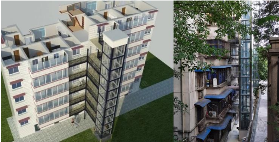
Figure 5.10: Outdoor lift installation, design diagram and example
