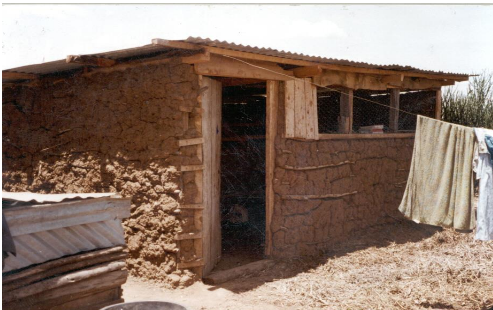
Photograph 3.6. A chicken house with iron roofing and mud walls as an adaptation of the housing intervention at a village in Ngarua-Laikipai region, Kenya
