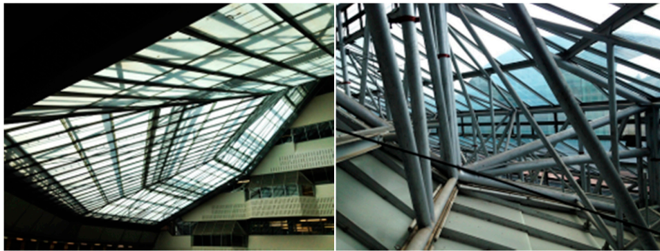
Figure 2. Glazed, double-skin roof of the library from inside the library (left) and inside the cavity (right).
