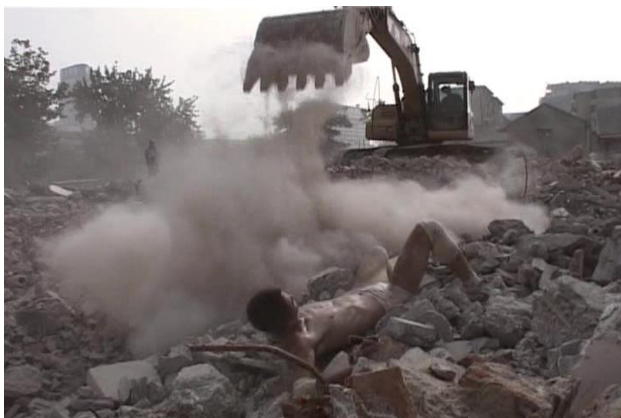
FIGURE 2.6: LI COMES INTO CONTACT WITH A FORKLIFT ON THE DEMOLITION SITE.
