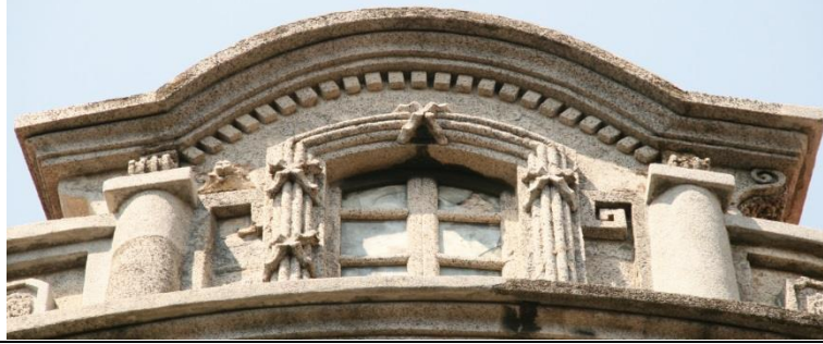
A- Fasces (a bound bundle of rods without an axe) framed window
