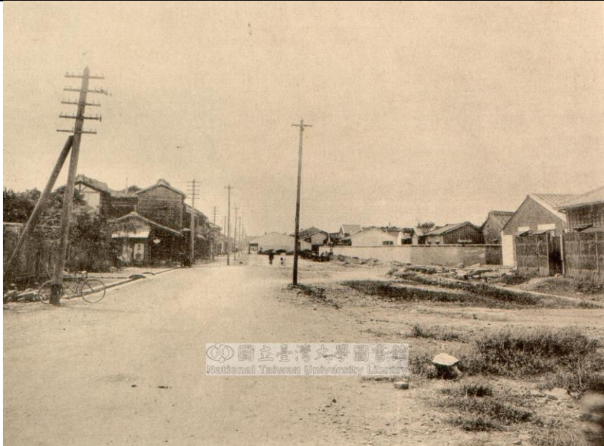
Fig.4.26- The Fu-hou Street before the urban redevelopment in Chengnei 439
