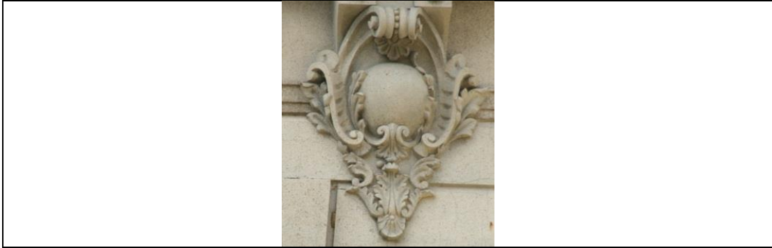
Fig.5.63- The residence of the Governor-General of Taiwan (1910-1912) 611
