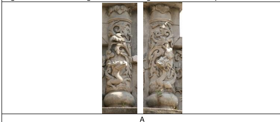
Fig.6.31-The motif of dragon columns on a gable in the Daxi shop-house
