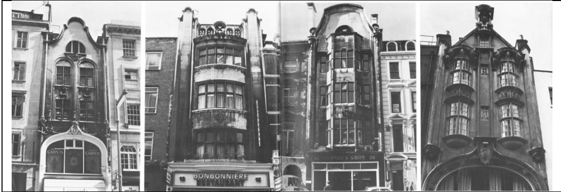
Fig.5.31- Shops and office buildings in London (c.1906) 536
