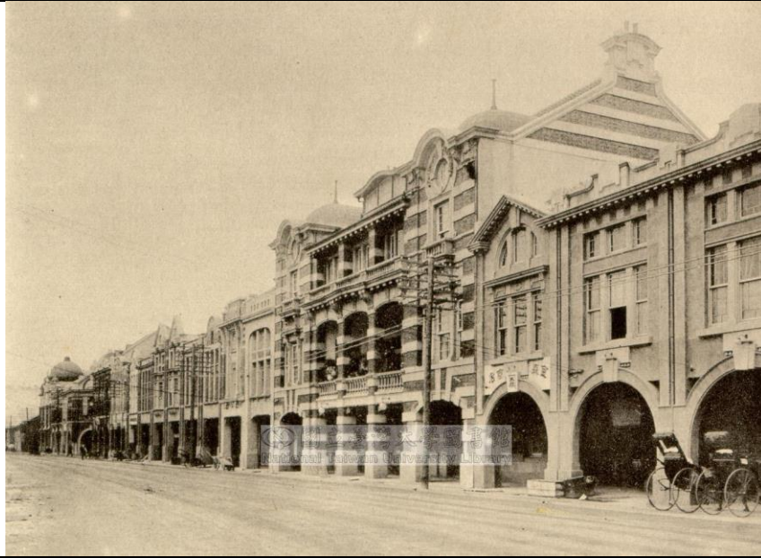
Fig.5.11- The shop-house in Chengnei (1912) 497
