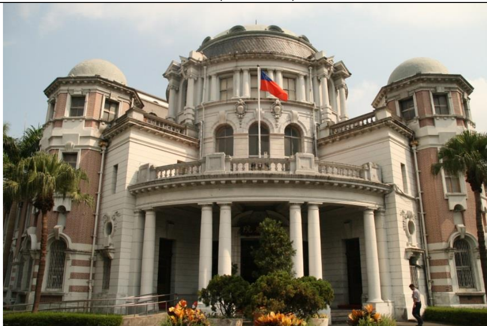
Fig.5.60- The Taihoku Prefecture Hall (1912-1915) 603
