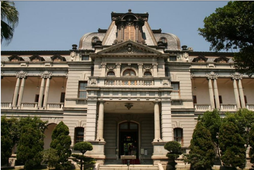
Fig.5.58-The residence of the Governor-General of Taiwan (1910-1912) 601
