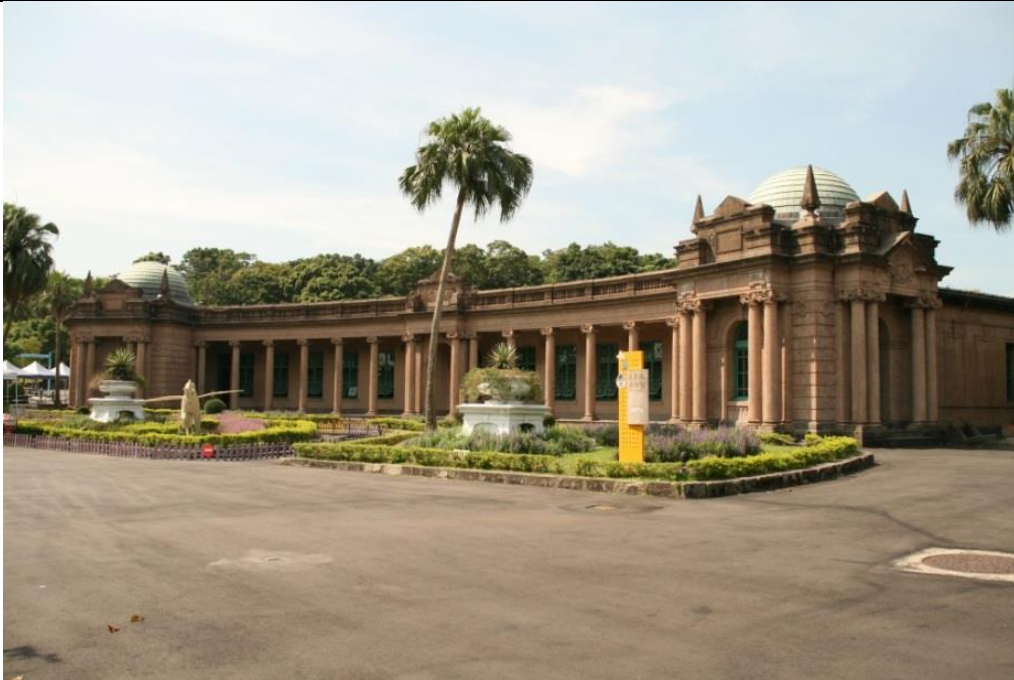
Fig.5.57- The Taihoku Pumping Station (1907-1909) 600
