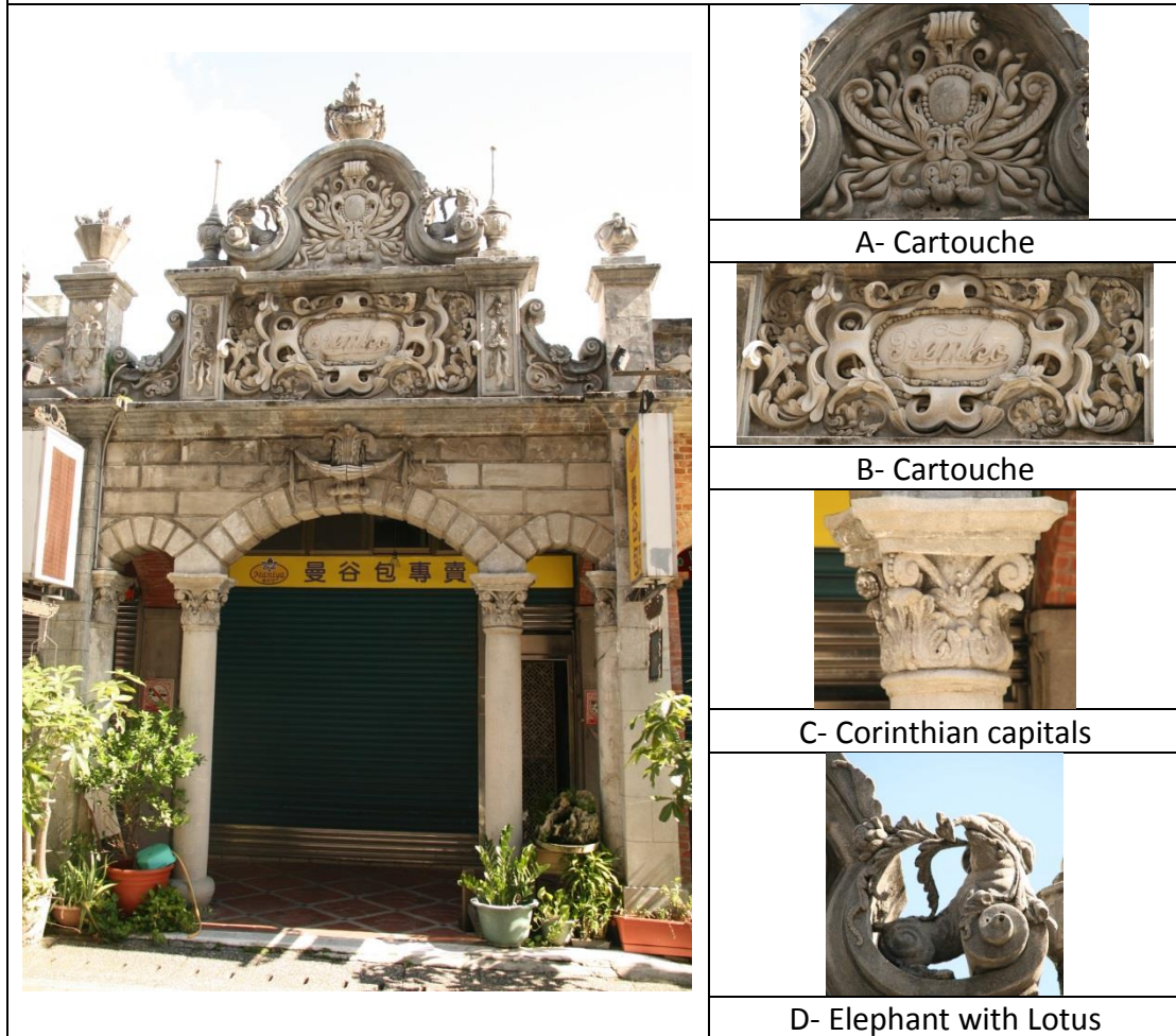
Fig.5.56- Shop-house in Daxi mixed with the motifs of the Taiwanese and the West 595
