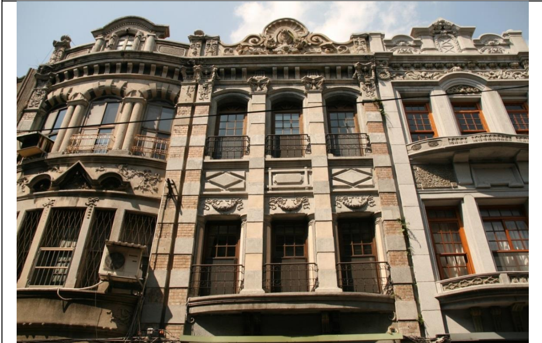
Fig.5.19- The shop-house in Dadaocheng (1920) 520
