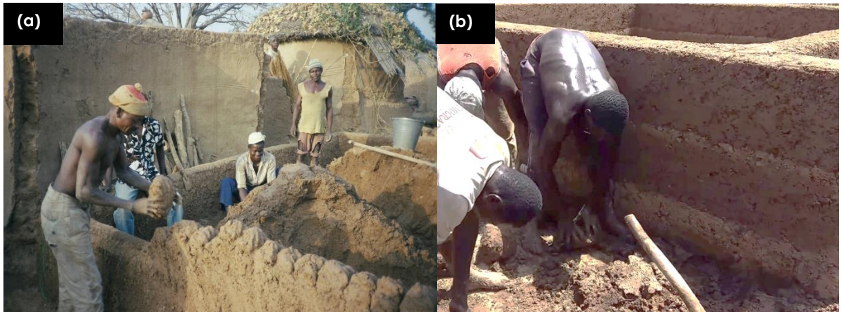
Figure 2-15: Cob technique, (a) shows how earth balls look when they are placed in the wall before they are pressed by hands, (b) shows how the final cob wall looks with all the layers,
