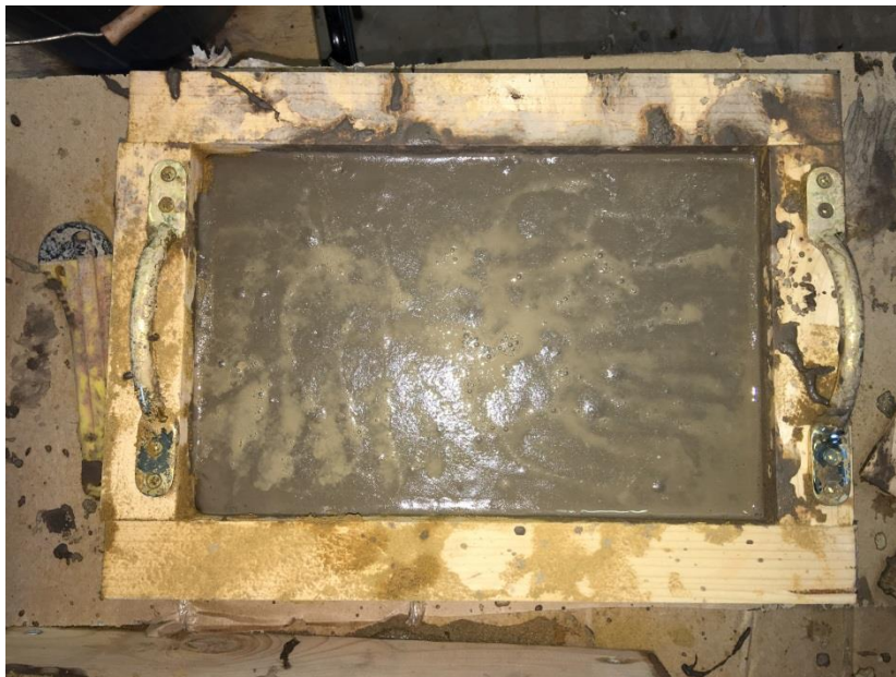
Figure 4-23: The levelled smoothed Sudanese adobe brick after scraping the excess mud and before removing the wooden mould
