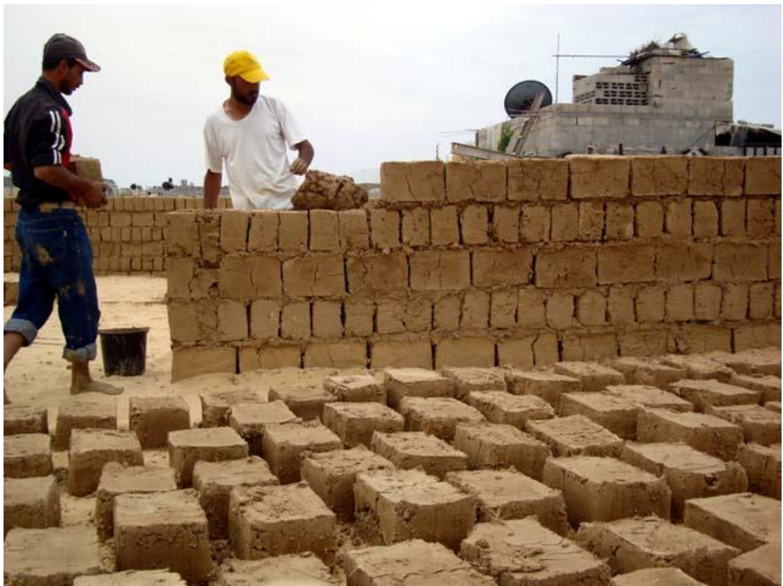
Figure 2-14: Adobe construction technique, Source: http://hopebuilding.pbworks.com/w/page/19229916/Denied%20steel%20and%20concrete%20Palestinians%20build%20mud%20brick%20homes%20in%20Gaza
