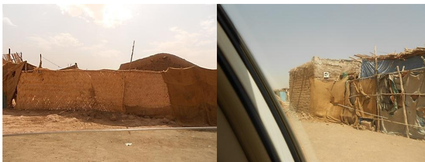
Figure 1-3: Simple houses built from the non-durable building materials (mud, sacks, carton and fabric) in the outskirts of Khartoum, Source: Author's collection, January 2013
