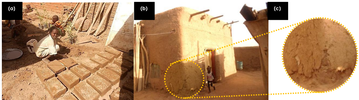
Figure 1-6: (a) Kids making adobe bricks during their summer school holiday and leave them on their bottom surface to start the drying process in the sun before turning them to their edges, (b) wall base eroded by the rain due to the absence of wall bases, (c) closer view of the erosion on the wall base
