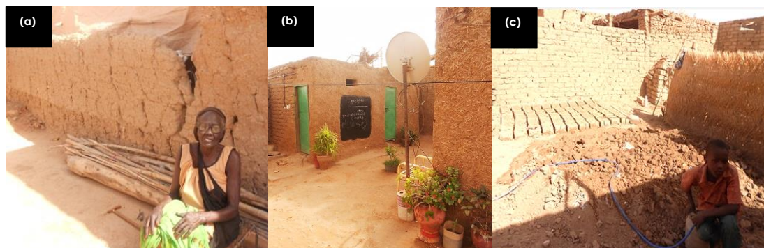
Figure 1-4: Earth houses in Khartoum urban areas, Sudan. (a) Cob wall (b) Adobe wall (c) Adobe brick making by young kids during their summer school holidays. Source: Author's collection, January 2013
