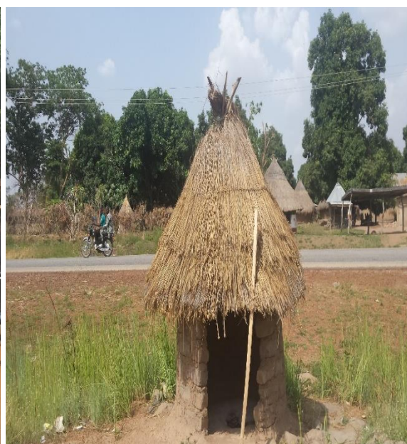
Figure 4.5: Communal latrine in Vandicom
