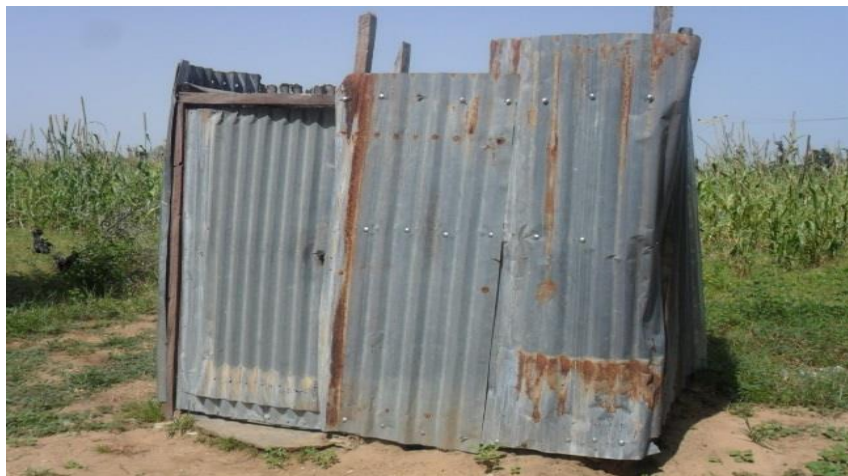
Figure 2.2: Latrine in Albarshi primary school, Kaugama LGA
