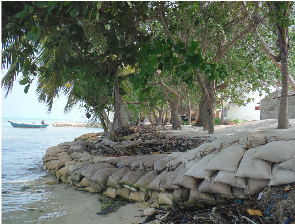
Fig. 4. Sandbags to mitigate coastal erosion.
