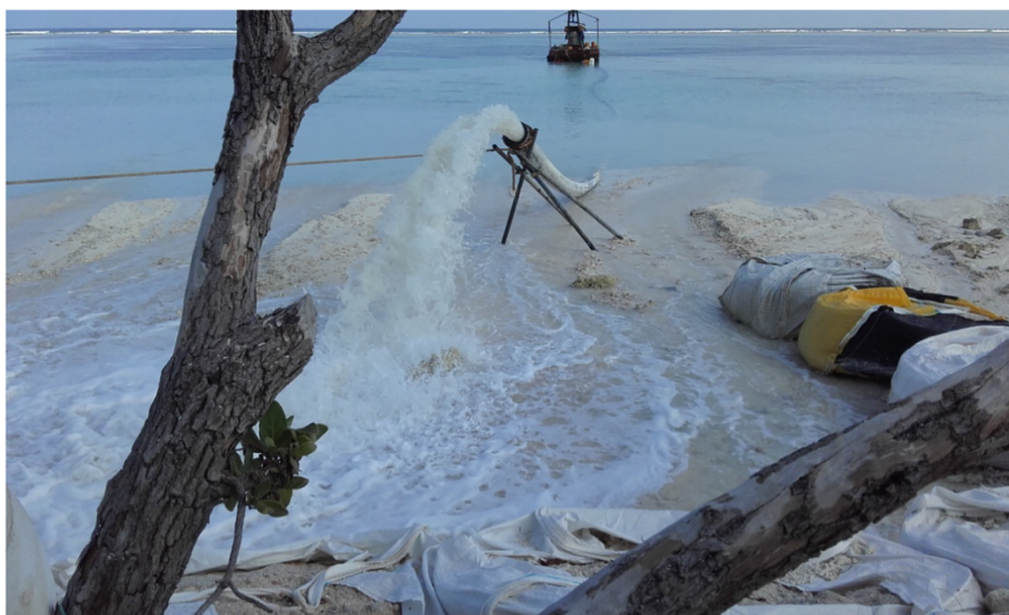
Fig. 2. Sand pumping for beach renovation.
