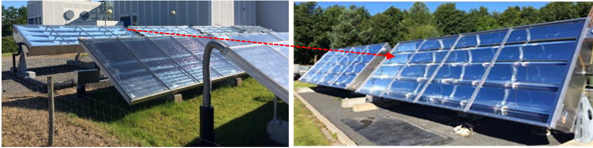
Figure 17 Compound parabolic trough collectors (Source: PolyCSP Aps/DTU)
