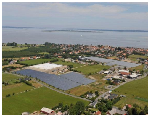
5a. Marstal plant (33300 m 2 )
