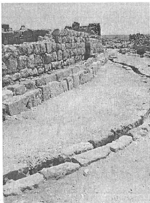
Fig. 7. Water-collecting channel at Shivta.
