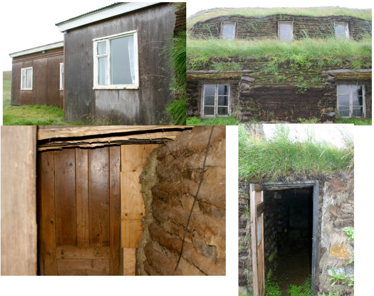
Figure 2.4. Galtastaðir, a turf house on a working farm in east Iceland, with glass windows, wooden doors and door frames, and a mid-20th century extension of wood and corrugated tin (top left). The home was occupied until 1967. Photos: Author's own.
