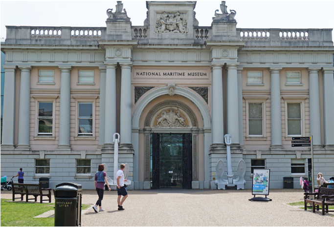
Fig 28. Anchors at the Stanhope Entrance to the National Maritime Museum
