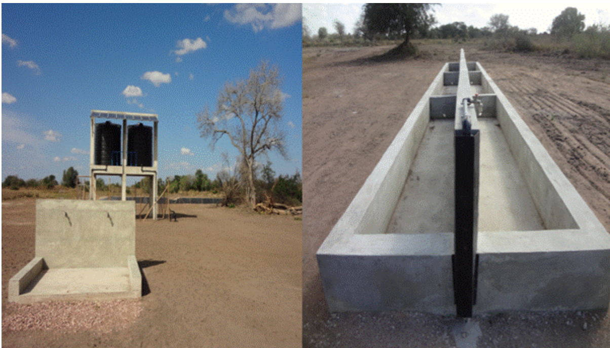
Water points supplied by the reservoir for human (left) and animal (right) consumption in Mbala-Vala, Guija (source: Author, July 2017)
