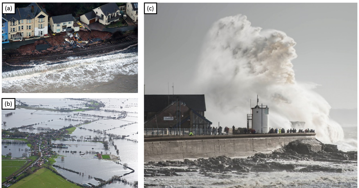
Figure 4.1: Images of storm impacts from DJF1314. (a) Breached sea defences and collapsed train line at Dawlish, Devon on 6 February 2014. (Source: Network Rail.) (b) The flooded Somerset Levels on 2 February 2014. (Source: Tim Pestridge.) (c) Large waves at Porthcawl, Wales on 5 February 2014. (Source: Karl Baker.)
