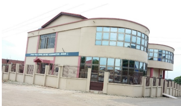
Newly constructed complex for Police office, library and ICT centre
