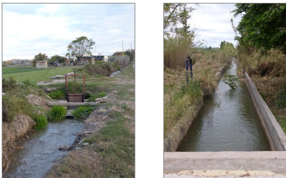
Figure 4.20 Earthen secondary channel (left) and lined channel (right) in Mendoza
