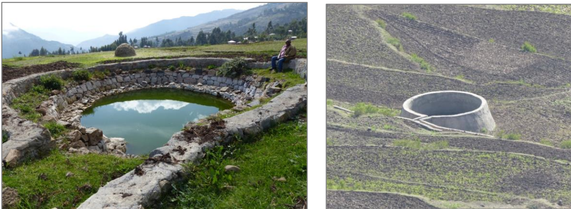
Figure 4.8 Traditional stone water reservoir (left) and concrete water reservoir (right) in Tsibet, Tigray
